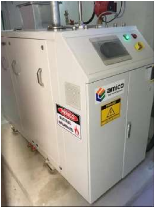
Fig. 6. Combinated Heating Power – CHP
